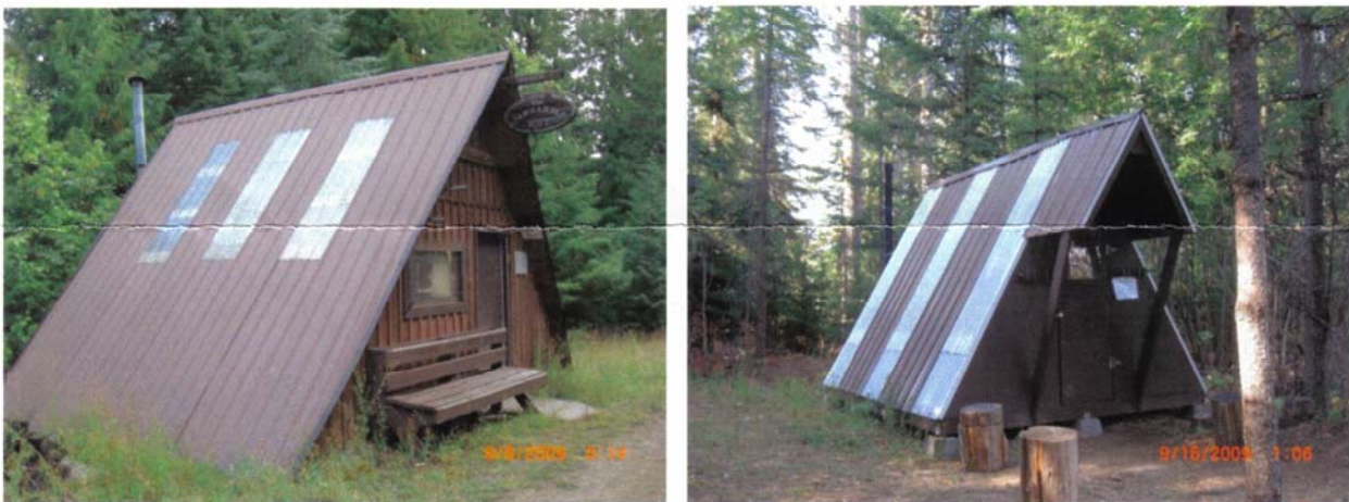
Figure 4. A-frame warming huts are in good condition, needing minor repairs.
