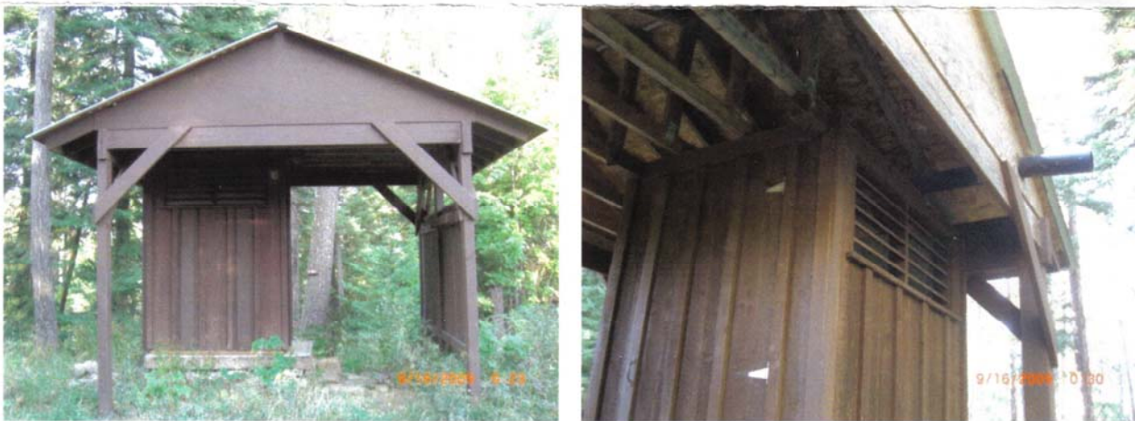
Figure 3. Wood-framed vault toilet and pavilion protecting it from heavy snow loads.
